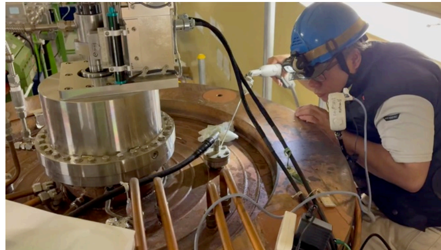
Solvent injected to the root of the monitor port
