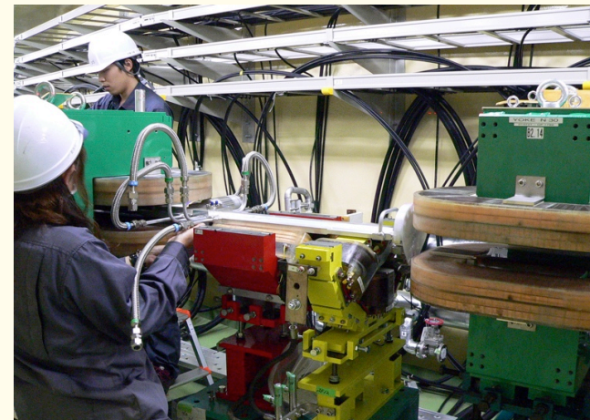
Installation of vac. chambers
