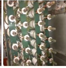
PCB capacitor replacement
