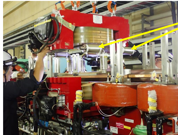
Wiggler magnet reassembly
