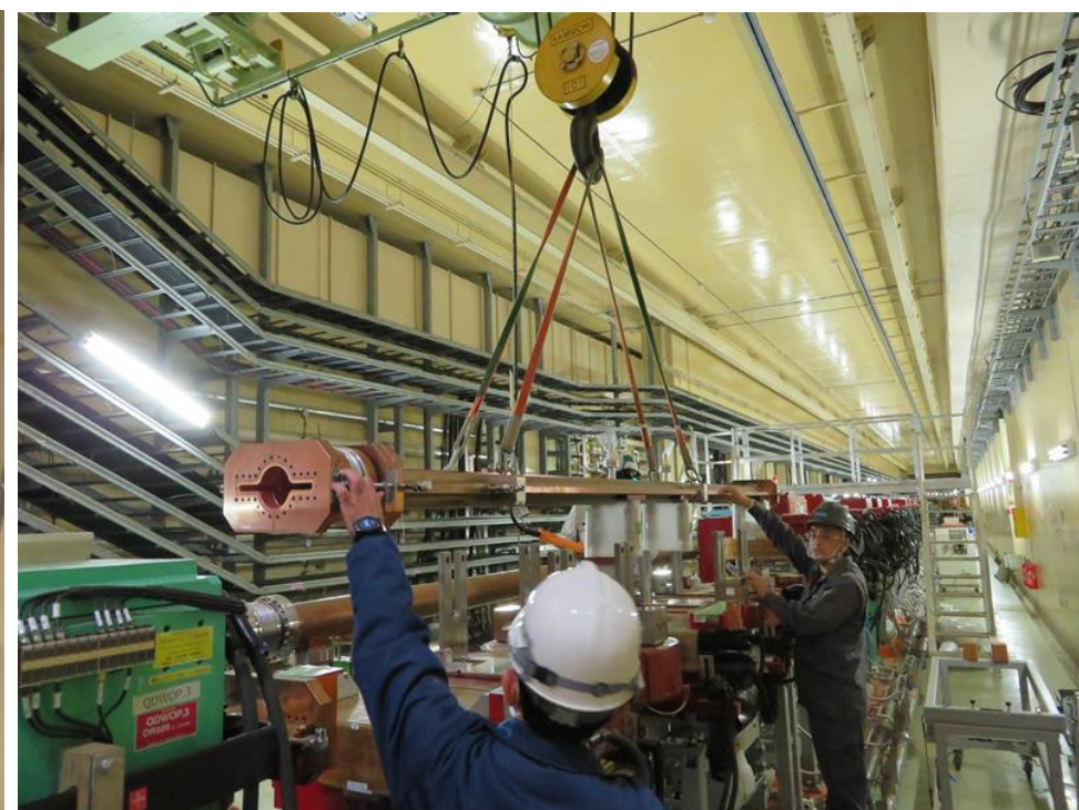
Wiggler beam pipe removal work
