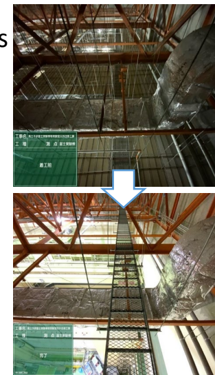
Ceiling aseismic reinforcing work
