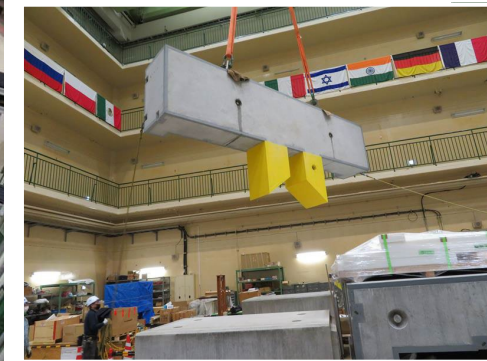
New concrete shields
