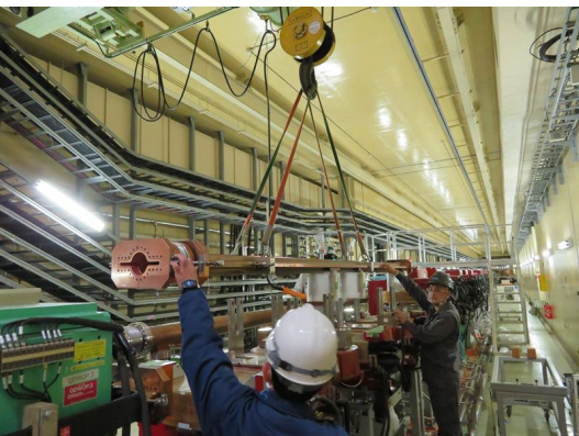
Wiggler beam pipe removal work
