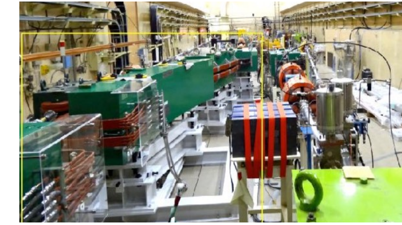
New energy compressor
