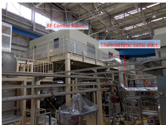
Figure 1: RF control room (outside view)
