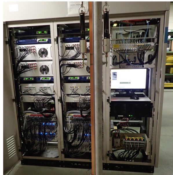
Figure 3: A photo of the standard unit for 4 quadrupole and 4 steering magnets.
