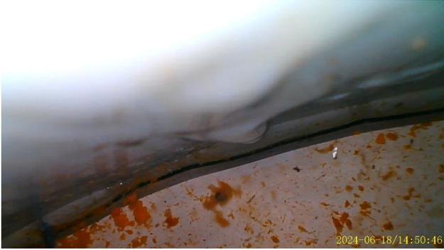
Figure 5: Water leak from klystron magnet
