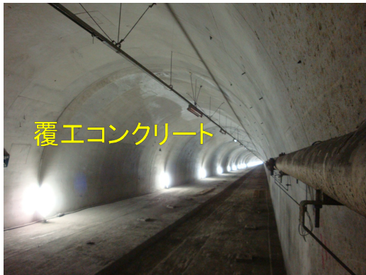
Photo 4: Inside view of D3 tunnel.
