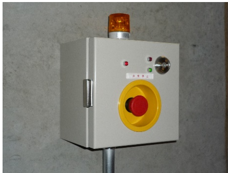
Photo 5: Switch which checks having evacuated.
