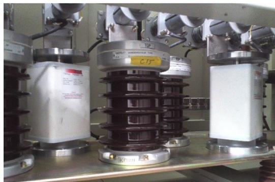
Figure 6: Mounted high voltage capacitors in a klystron modulator. Rectangular ones are new capacitors made by NWL CAPACITORS. Others are original ones.
