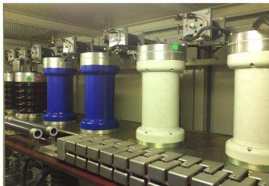
Figure 5: Mounted high voltage capacitors in a klystron modulator. Four capacitors in the front side are used capacitors transported from AIST. Two capacitors in the back side are the original capacitors used in this modulator.
