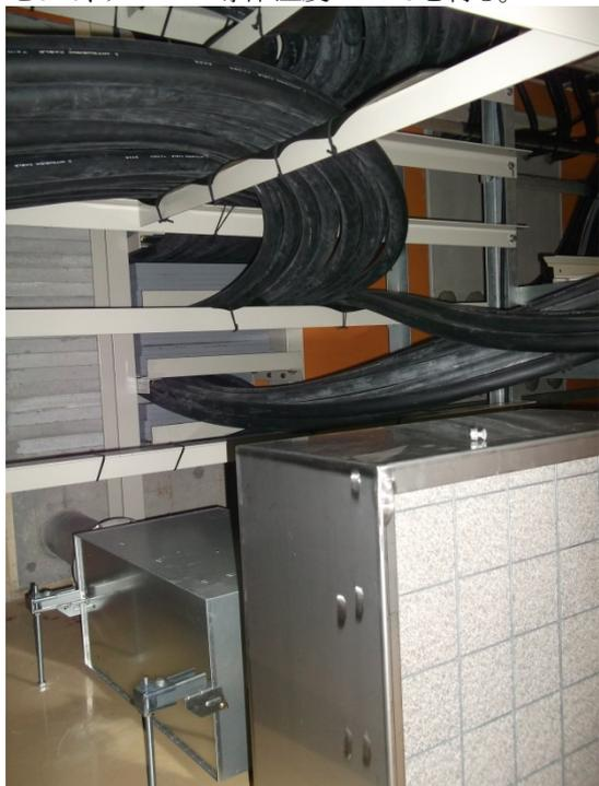
Figure 4: Cable cooling system with FDF.
