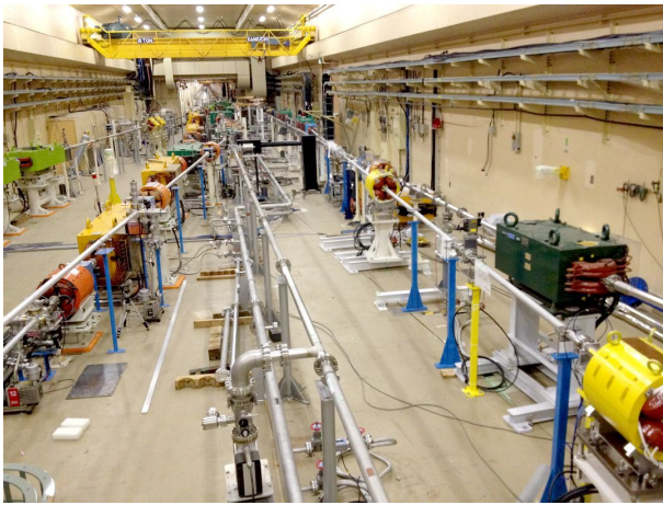
Figure 5: The beam switch yard at the end of linac. From right to left, beamlines of PF, PF-AR, straight dump, SuperKEKB LER, HER, and east dump.
