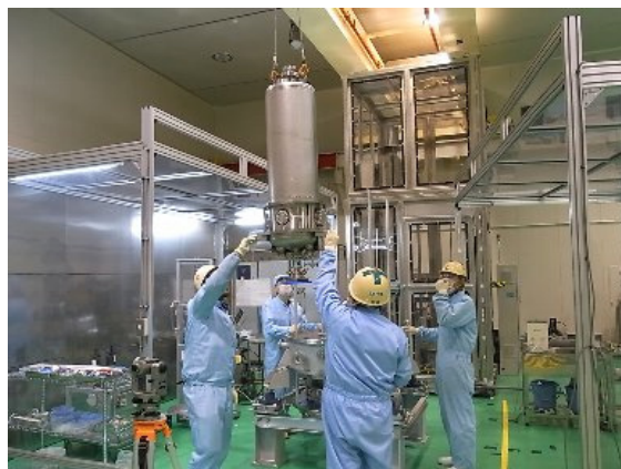
Figure 8: Heavy parts are brought into clean room using crane. Workers are wearing ISO7 clean ware.
