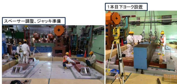
Figure 5: Alignment of the bottom yokes.
