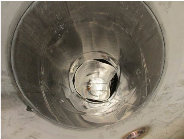
Figure 11: Dented magnetic shield inside the vertical cryostat after the trouble.
