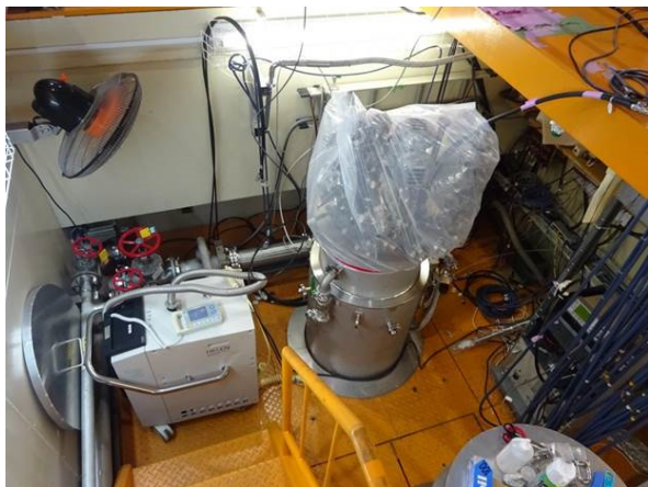
Figure 8: He leak check of the vertical cryostat by hood method.
