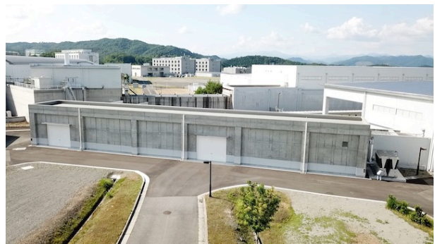
Figure 4: Bird view of new building.
