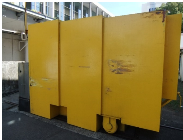
Figure 5: Photo of radiation shield doors.
