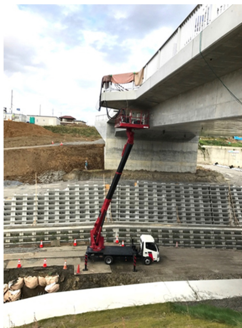
Figure 7: The photo of Bridge NDT with 3.95 MeV Linac.
