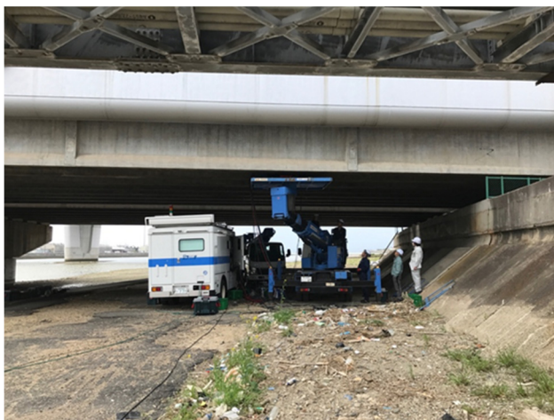
Figure 9: The photo of Bridge NDT with 950 keV Linac.
