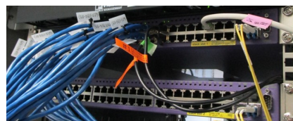
Figure 4: Edge switches.
