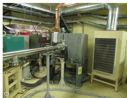
Figure 5: The beam dump at the positron dump ring injection line.
