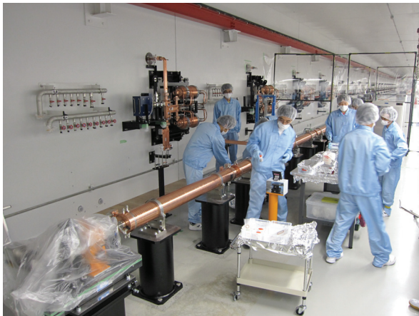
Figure 5: View of assembly of Vacuum Components
