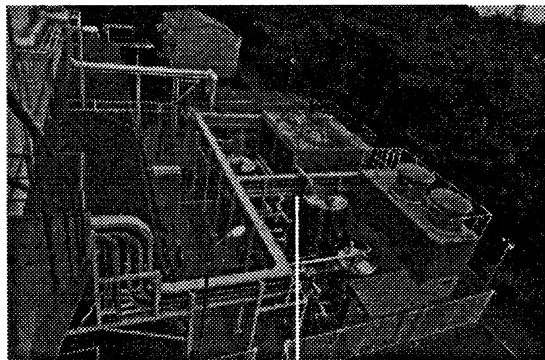
(C) Cooling tower
